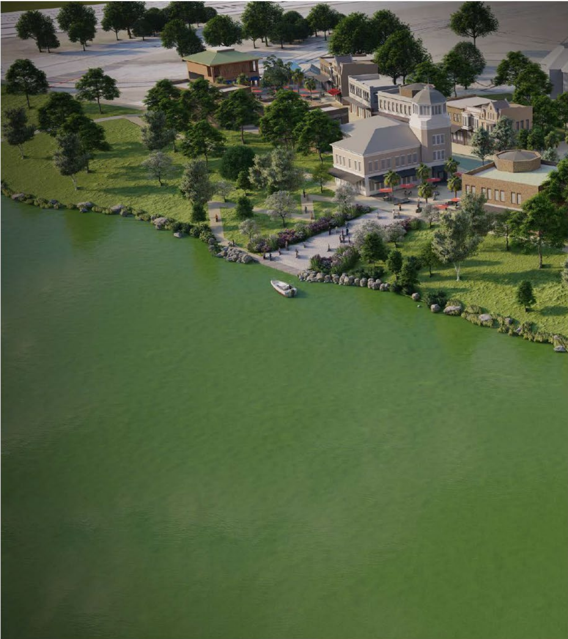
Aerial view of the Waterfront
