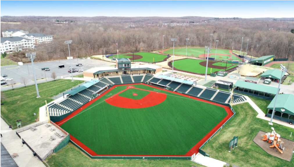
A ballfield in Aberdeen, Maryland.
