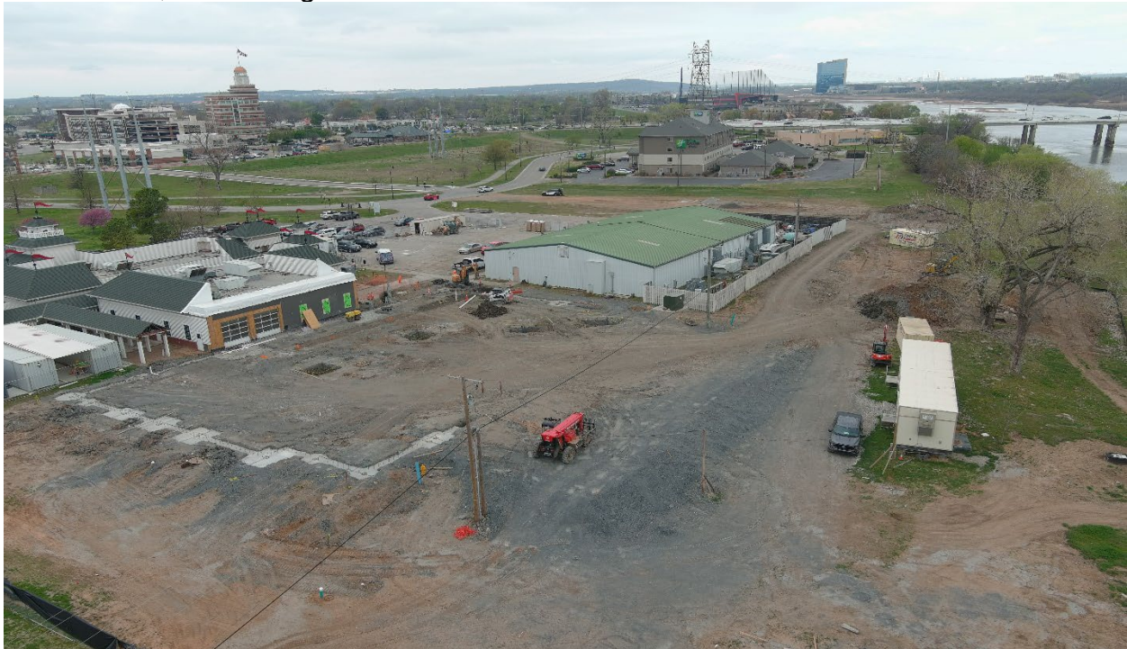
AQUARIUM CONSTRUCTION PROJECT
