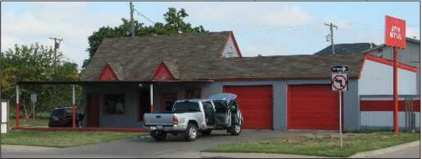
Figure 5: Old photo site.
