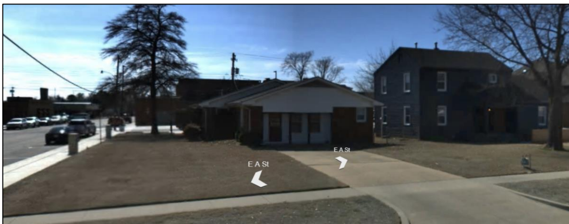
Figure 4: View of black house/office to be torn down for new project.
