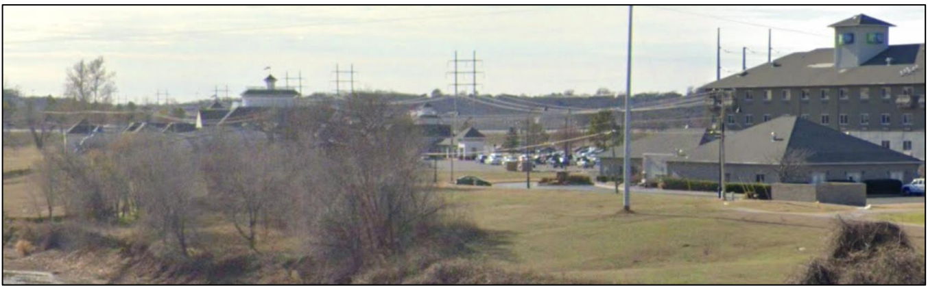
Figure 6: Site from Main Street Bridge
