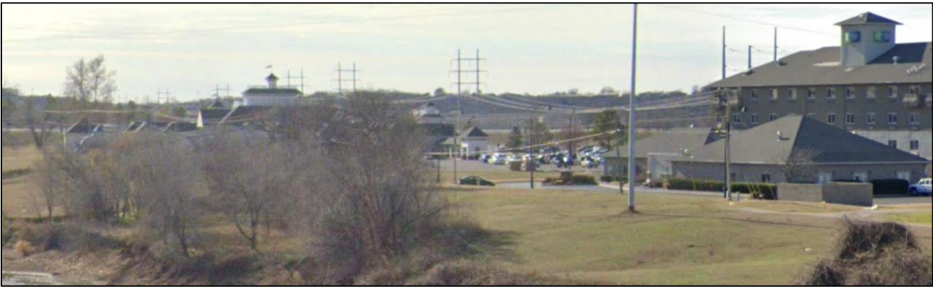
Figure 6: Site from Main Street Bridge
