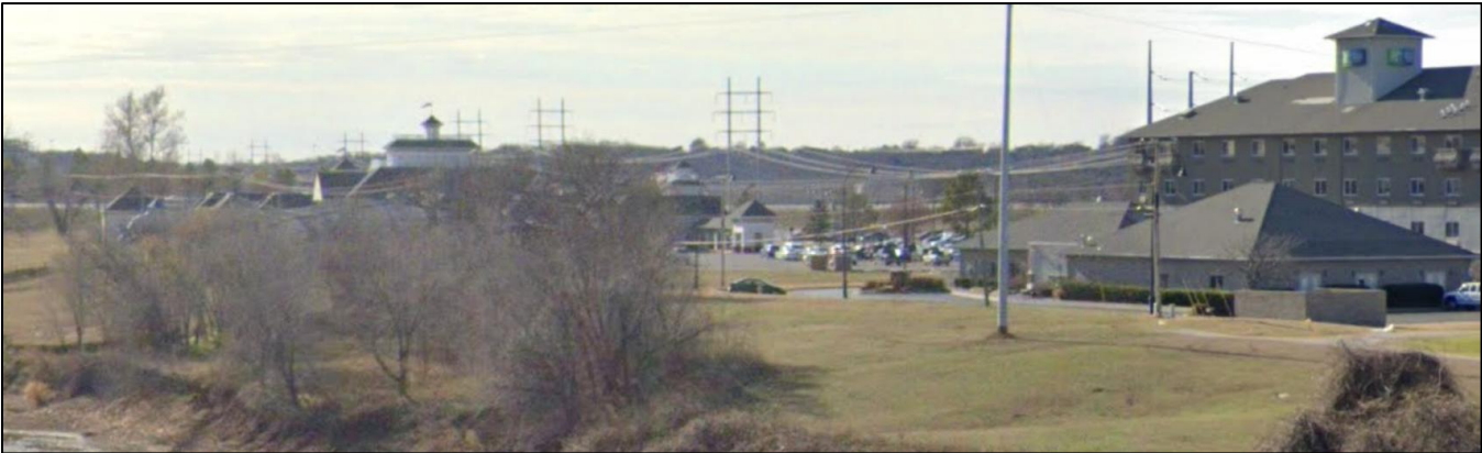
Figure 6: Site from Main Street Bridge
