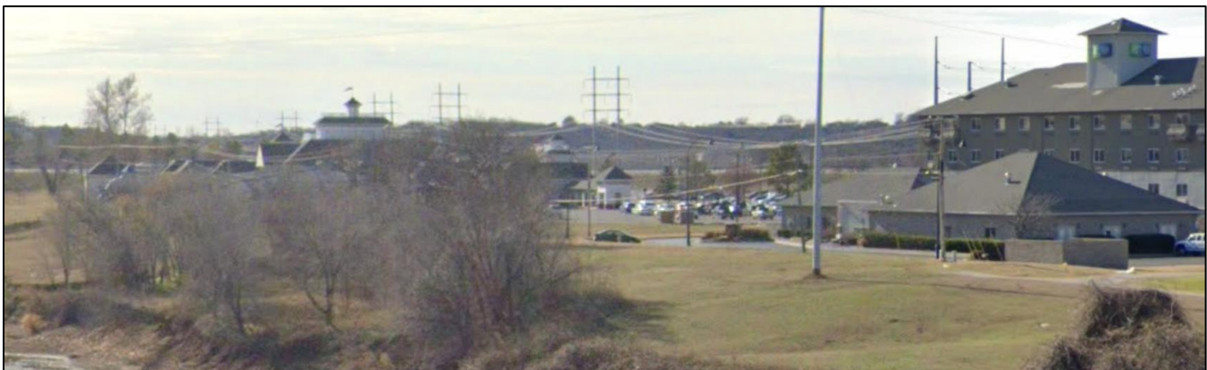
Figure 6: Site from Main Street Bridge
