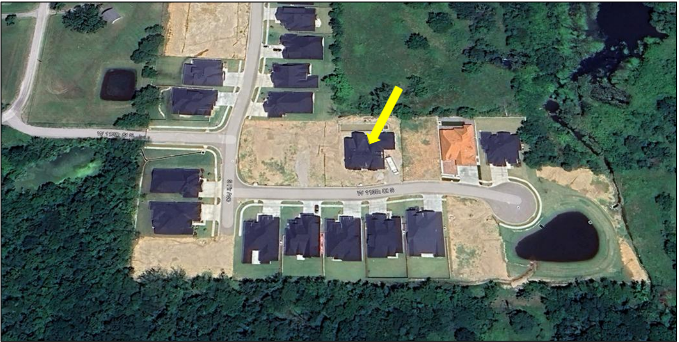
Figure 2: Google Earth Photo so subject house.
