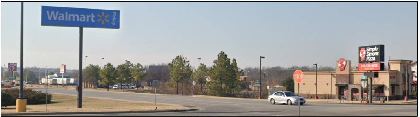
Figure 19: Glenpool Walmart Subdivision | pole signs
