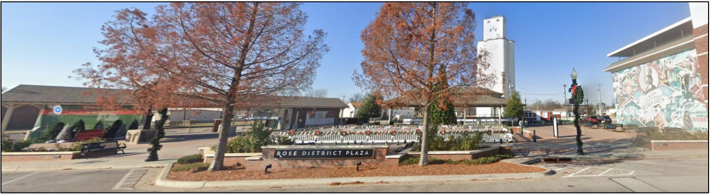
Figure 28: Broken Arrow Main Street | Monument sign
