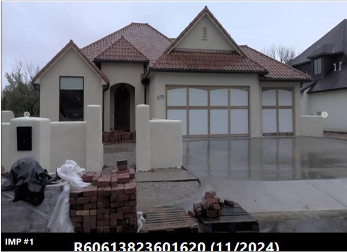
Figure 5: image from Assessor data during construction
