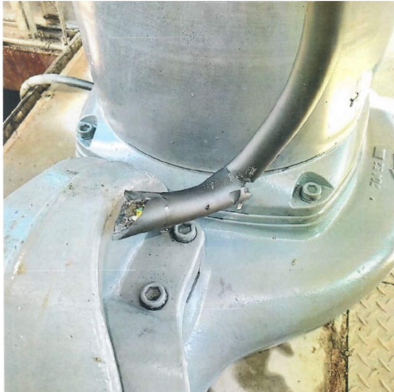
Float Ingested into Influent Pump 1
