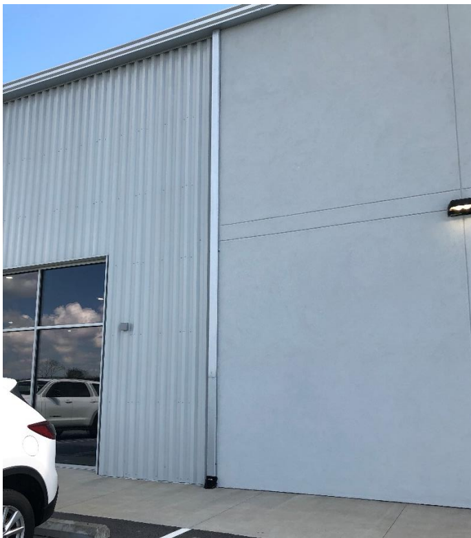
East of Front Door Showing Stucco and Metal Panel
