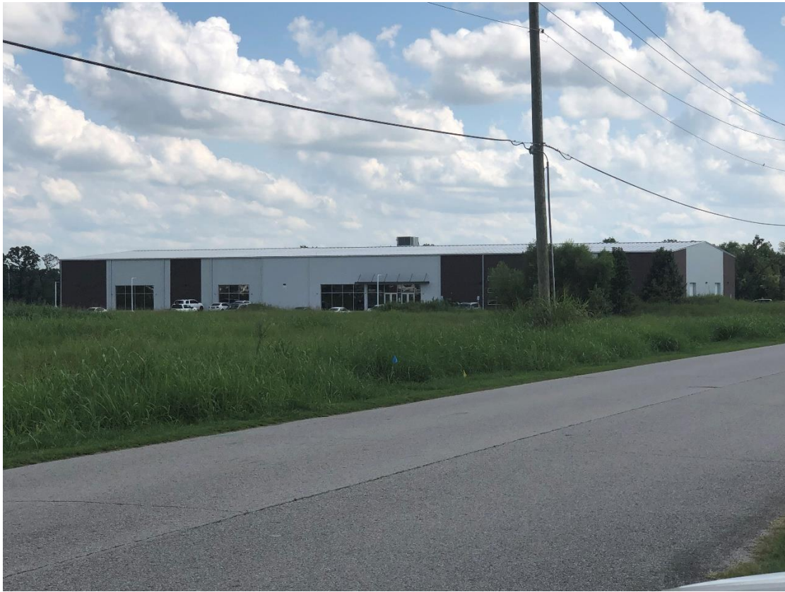
North Elevation Facing Main Street
