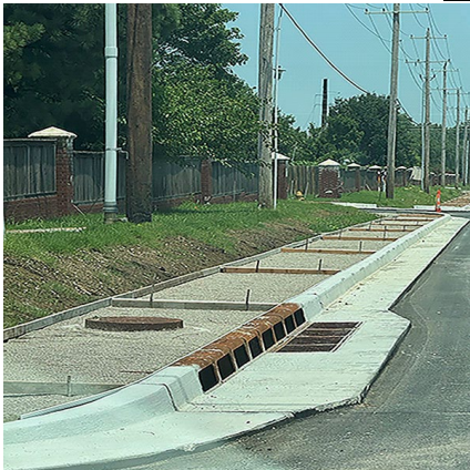
Framing of sidewalk – Framing of ADA compliant sidewalk on the westside of Elm Street to facilitate the movement of pedestrian traffic.
