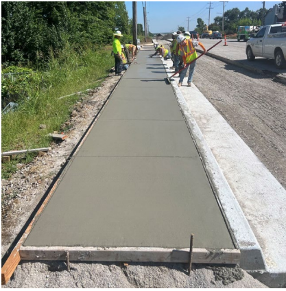
Sidewalk westside of Elm Street – Concrete placement of ADA compliant sidewalk on the west side of Elm Street.
