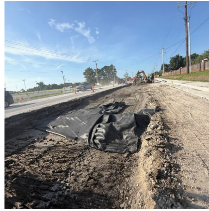
Westside of Island #2 Fabric and Agg – placement of Terratex fabric and aggregate base in preparation of asphalt for the widening of Elm Street.
