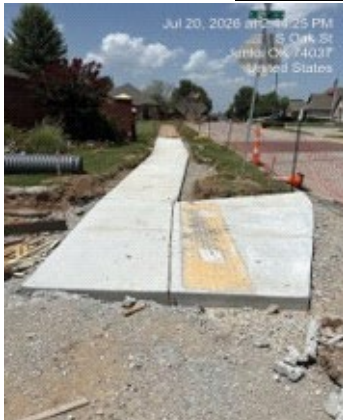
West connection to existing sidewalk at S. Oak St.
