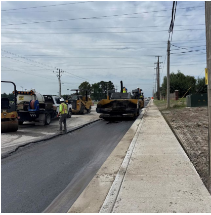
Island #2 (Westside) - Placement of asphalt to the west of Island #2.
