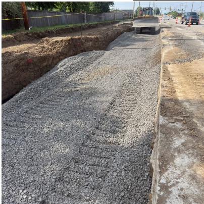
Elm Street Widening (Eastside) - Placement of TerraTex fabric for subgrade stabilization and installation of aggregate base for roadway. Aggregate base is tested for compaction and verification of grade prior to the placement of asphalt.
