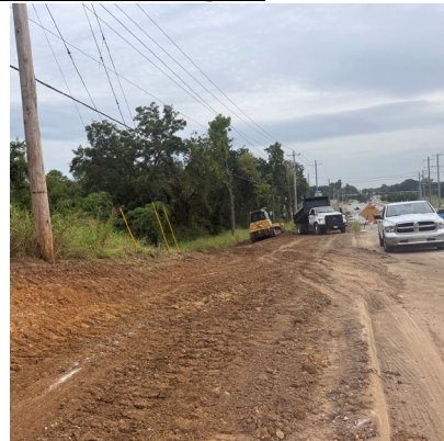
Elm Street Widening (Westside) - Excavation for roadway widening on the westside of Elm north of The Goddard School. This area will be tested for compaction and stability prior to aggregate placement for roadway.
