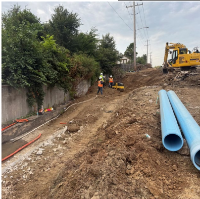
Waterline A - Installation of Waterline A between 112th and 114th on eastside of Elm Street.
