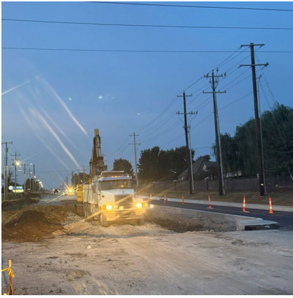
Elm Street Widening (Eastside) - Excavation prior to installation of aggregate base for roadway. Aggregate base is tested for compaction and verification of grade prior to the placement of asphalt.
