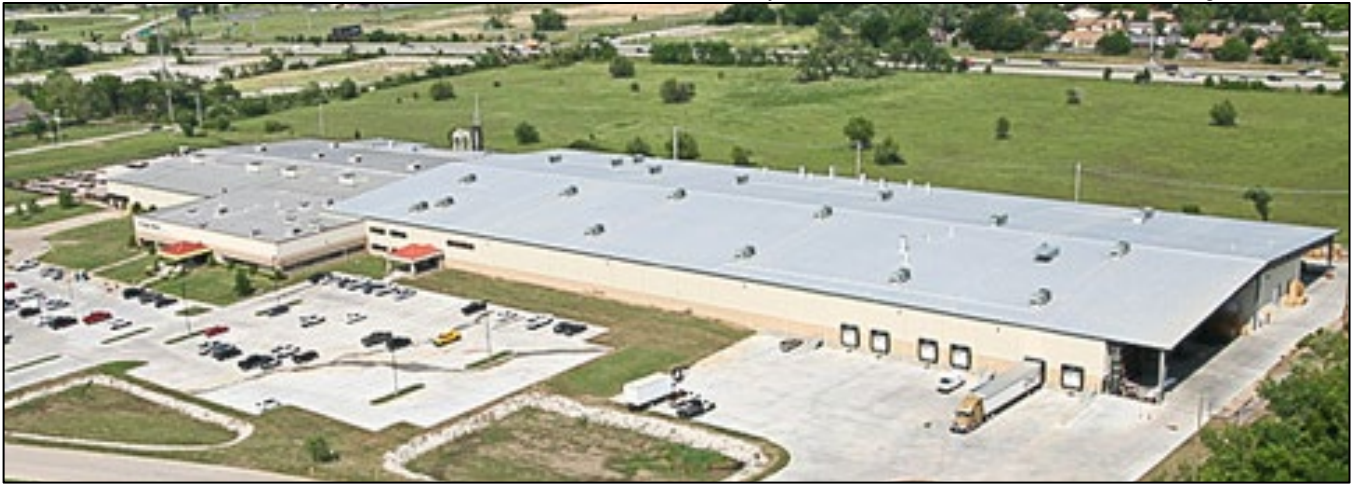
Figure 2: TWG Dover Aerial View from East (back side)
