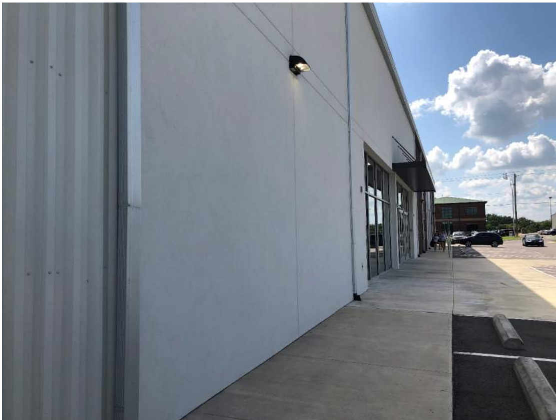
Front Door Area Looking West
