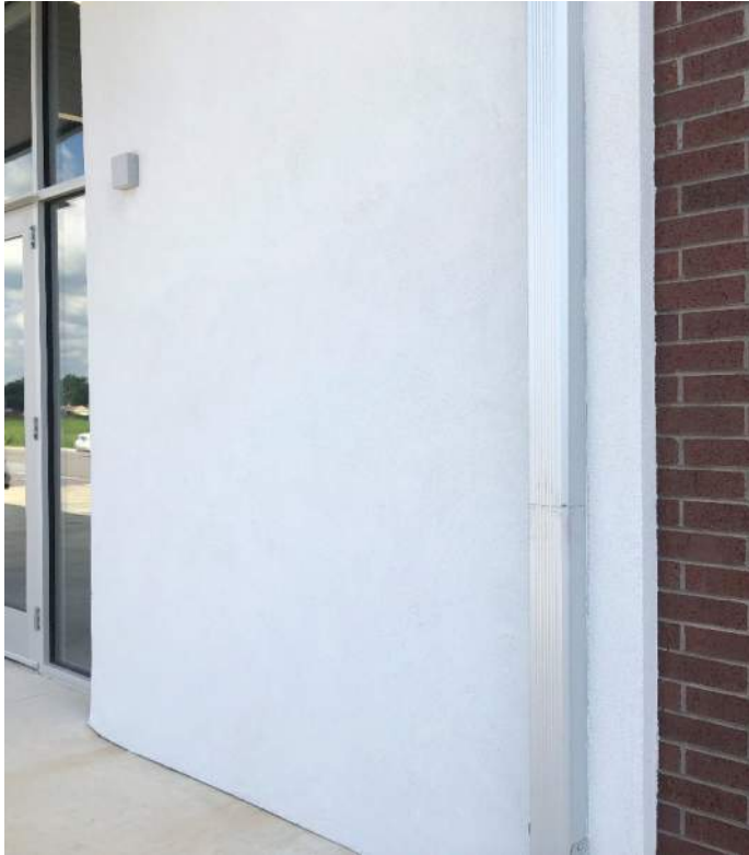
West Side of Front Door
