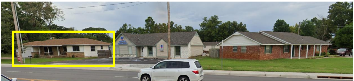
Figure 2: View of Residential Structure from east.
