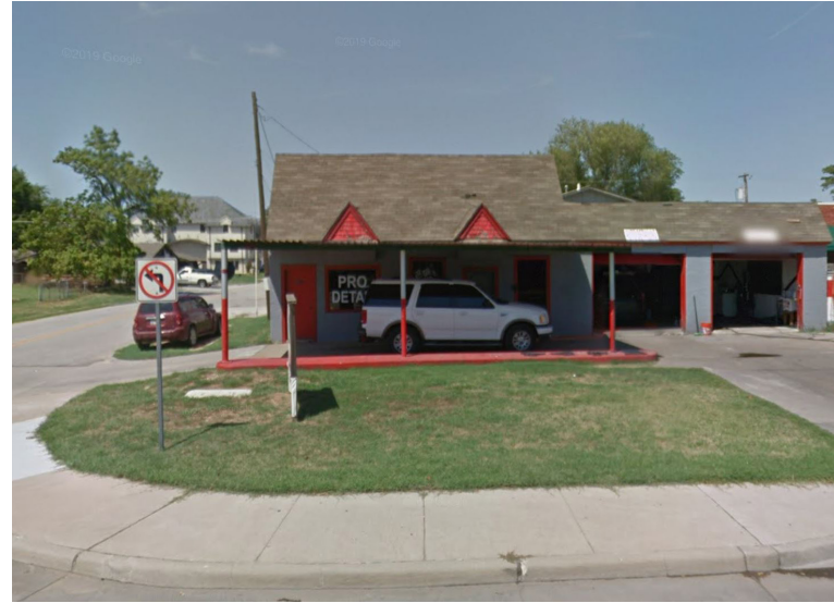
Facade Improvement - Before
