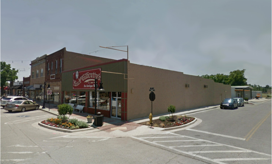
Utility Line Burial - After
