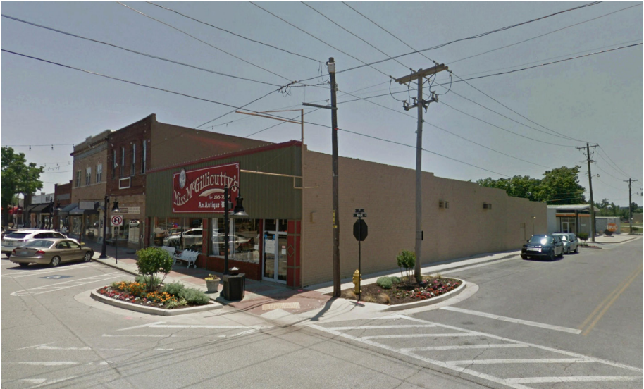
Utility Line Burial - before
