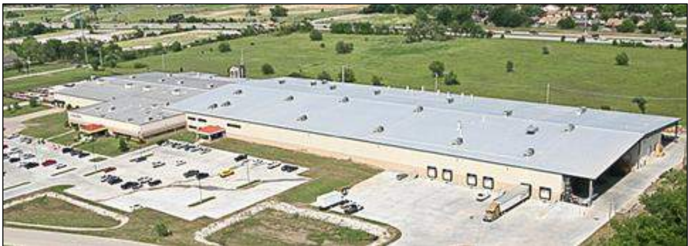
Figure 2: TWG Dover Aerial View from East (back side)
