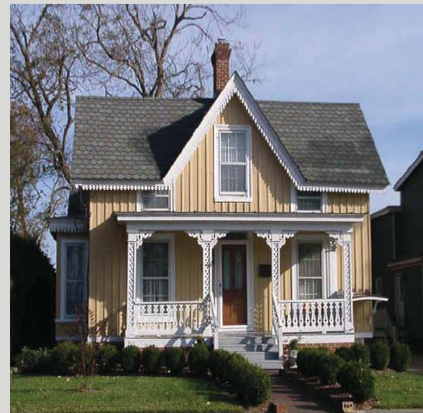
EARLY 1900s - BOARD & BATTEN SIDING
