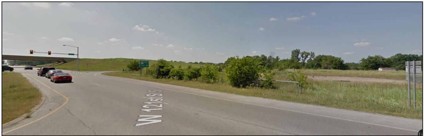
Figure 4: View of Lot from the south
