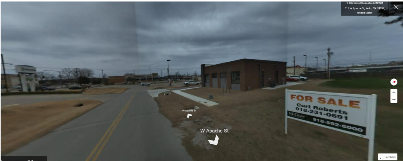
Figure 4: Web image of facing west. (W. Apache St. is Aquarium Place)
