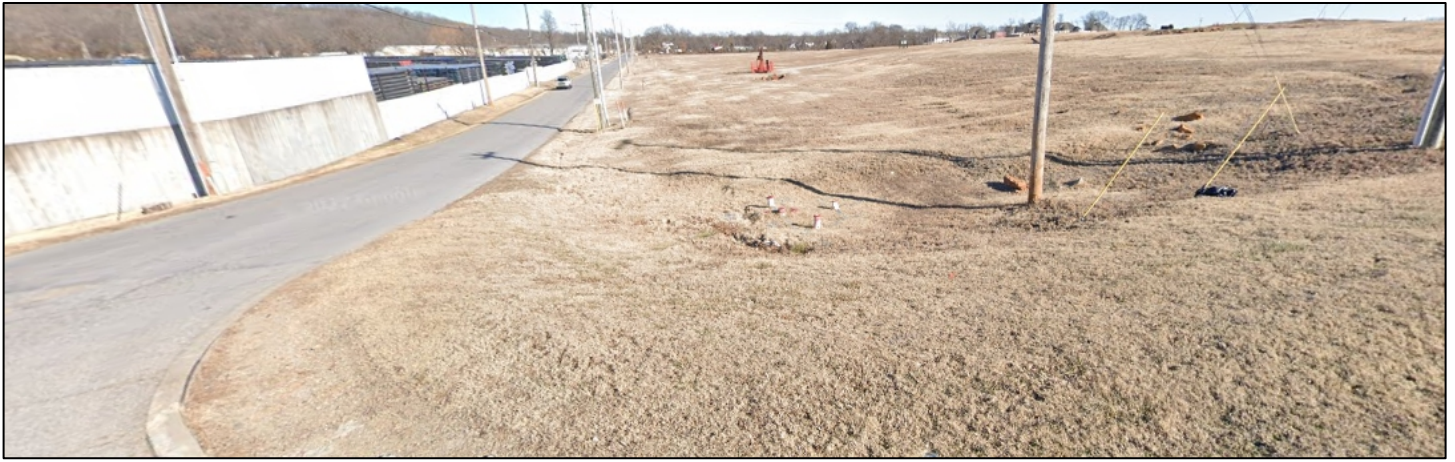
Figure 7: Google Earth view of 33 rd W. Ave looking north
